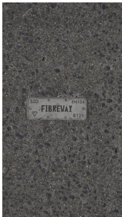
Manhole covers around Telehouse. They mark the places where the fiber enters the complex, and there are hundreds. Mostly UK/ US telecomms companies. Some of the names have been deliberately gouged out following corporate takeovers. Brand identity is real. 2 June 2019
