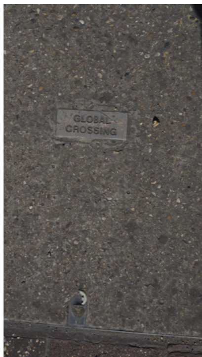
Manhole covers around Telehouse. They mark the places where the fiber enters the complex, and there are hundreds. Mostly UK/ US telecomms companies. Some of the names have been deliberately gouged out following corporate takeovers. Brand identity is real. 2 June 2019
